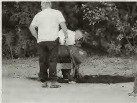
Highway Personnel make Repairs to Town Hall Parking Lot.
